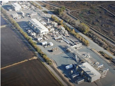
Photo courtesy of https://www.conservation.ca.gov/calgem/PublishingImages/Natural-gas-storage-facility.jpg
